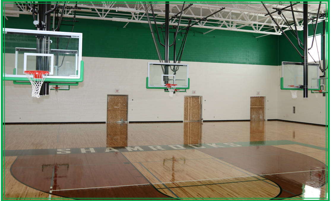
The installation of the 22,000 square foot gym floor has been completed.
