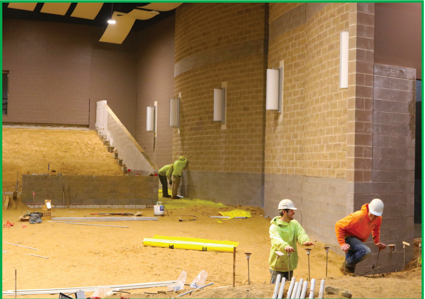
The auditorium, which will seat 750 people, is currently under construction.
